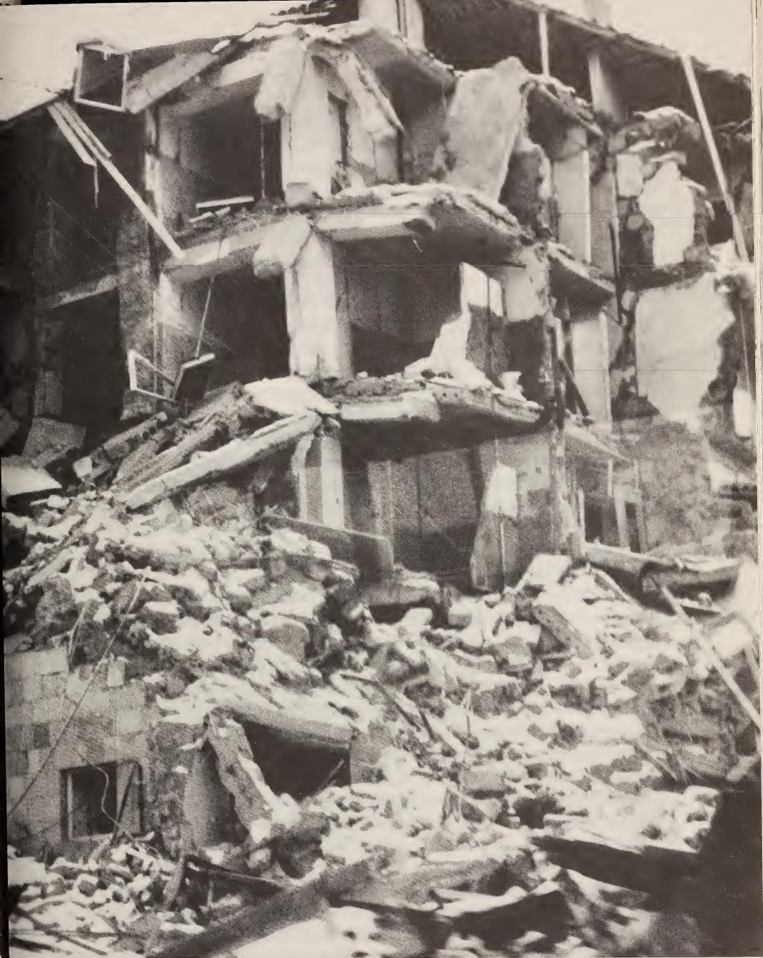
*Apartment house in Spitak, Armenian Republic, destroyed by an earthquake in December 1988 that registered 6.9 on the Richter scale. Such apartment houses were not designed, or built, to withstand seismic activity of that magnitude. The earthquake claimed 25,000 victims. Courtesy United States Geological Survey*
